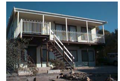
View of house from rear.
